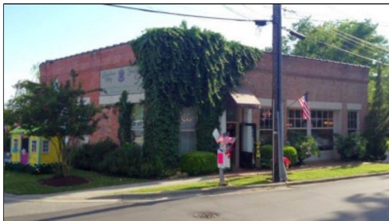
300 Water Street today.
