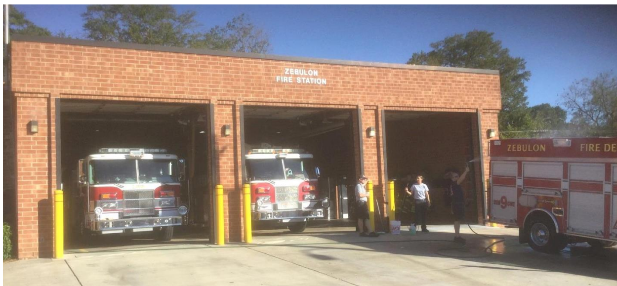
Figure 40 - First Out Apparatus During Daily Inspection
