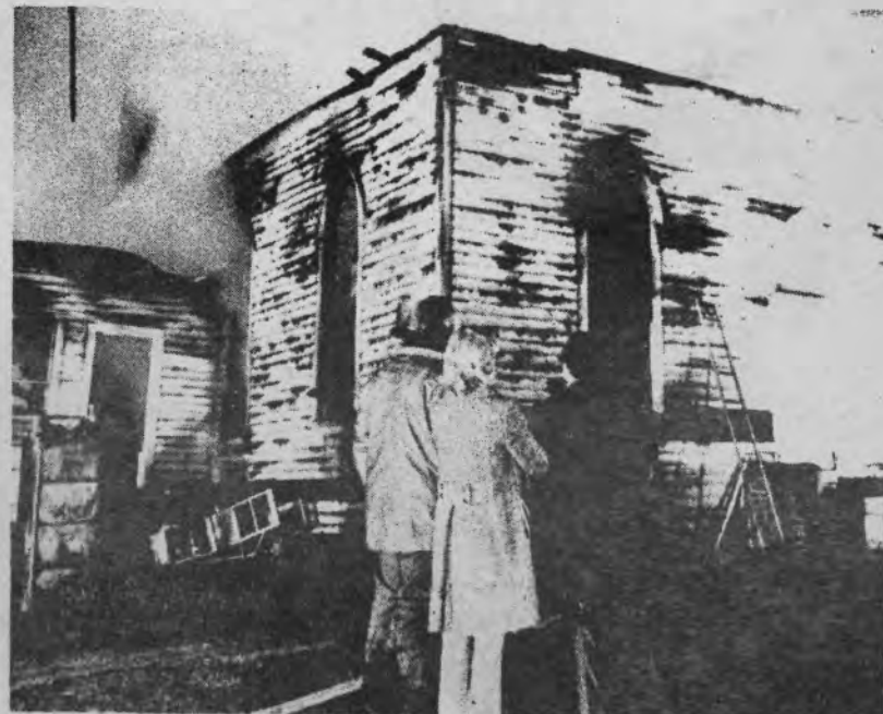
UP IN SMOKE - Garner's historic Town Hall went up in smoke and flames between 12:30 a.m. and dawn recently. The extra heavy roof on the structure collapsed within minutes after firemen arrived on the scene. After the collapse, the firemen concentrated their efforts on hosing down the water tower to keep the intense heat and flames from buckling the legs.
