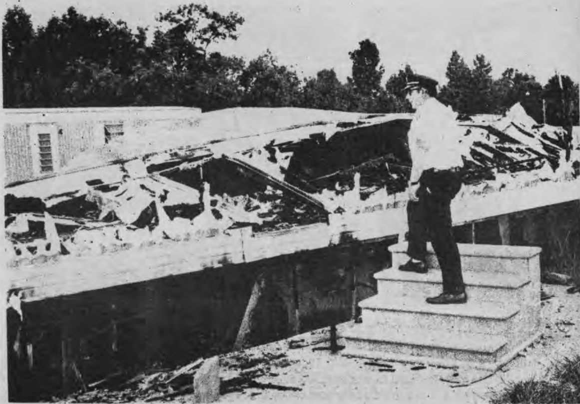
Capt. H. T. Link of the Statesville Fire Department, surveys a mobile home destroyed by fire which might have been contained if a smoke detector had been in use.
