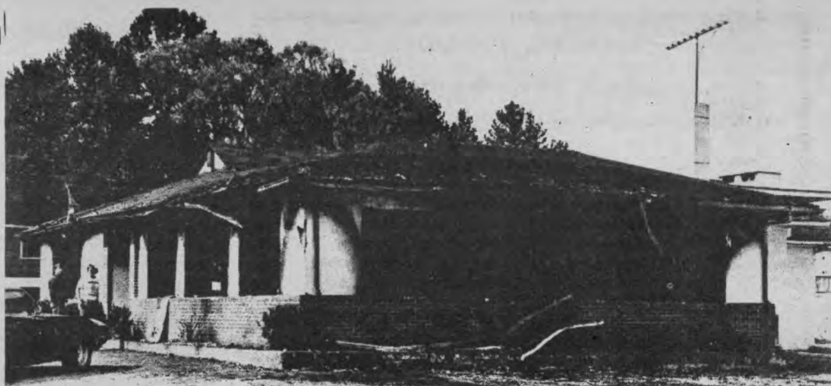
This is the fire-gutted building on West Lebanon Street housing the Hot Rod Barn. Cause of the early morning blaze is undetermined.
