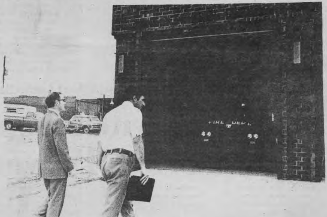
Making final inspection
