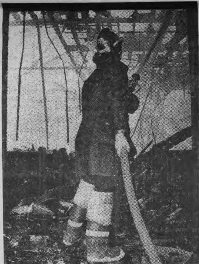
GUTTED EDGEWOOD BAPTIST CHURCH Asheville Citizen Photo
