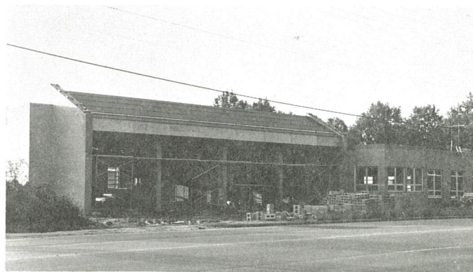
New Bethesda Station Under Construction
