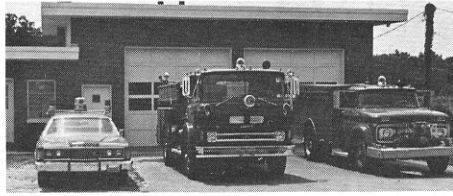
Station No. 27 McLeansville Fire Department
