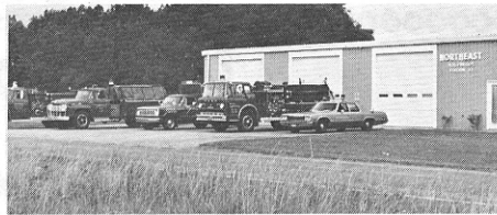
Station No. 32 Northeast Fire Department
