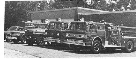
Station No. 18 Deep River Fire Department
