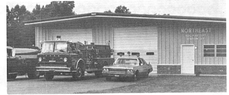
Station No. 33 Northeast Fire Department
