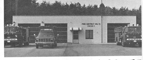
Station No. 5 Fire District 13
