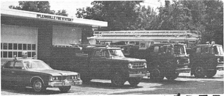
Station No. 7 McLeansville Fire Department
