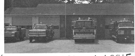
Station No. 14 Fire District 14
