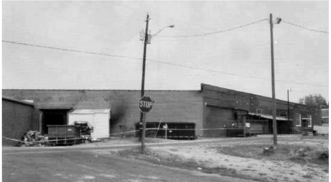
View of the south end, the southeast corner, and the front of the Imperial Foods building.
