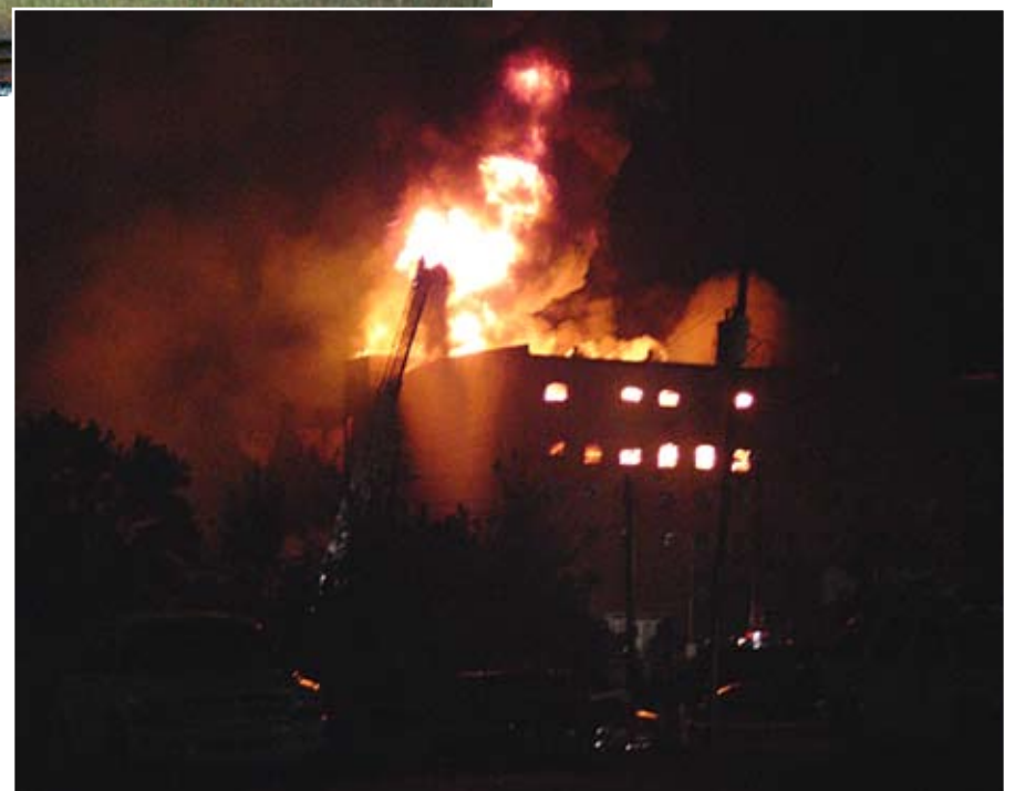
Firefighters continued to fight the blaze through the night; one fire engine narrowly escaped damage when the west wall of the building collapsed around daybreak.
